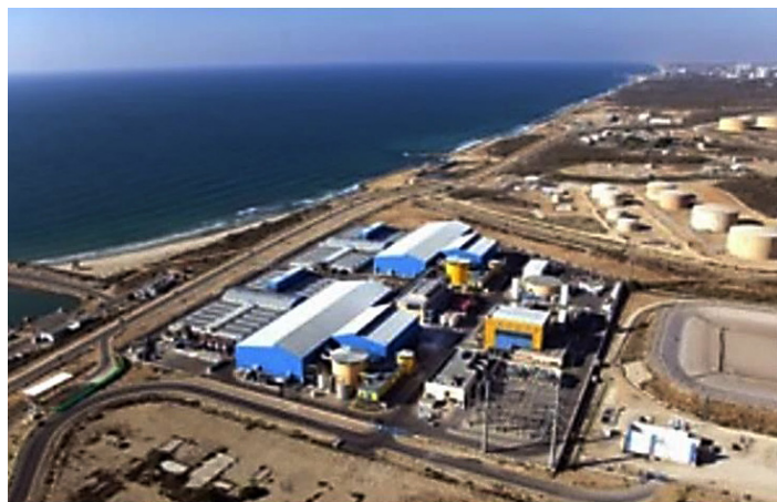
Figure 7: The Ashkelon Desalination Facility produces about 5 percent of Israel's total water needs.
